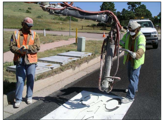
City Traffic Engineering crews mark a bike lane on a newly resurfaced City road.
