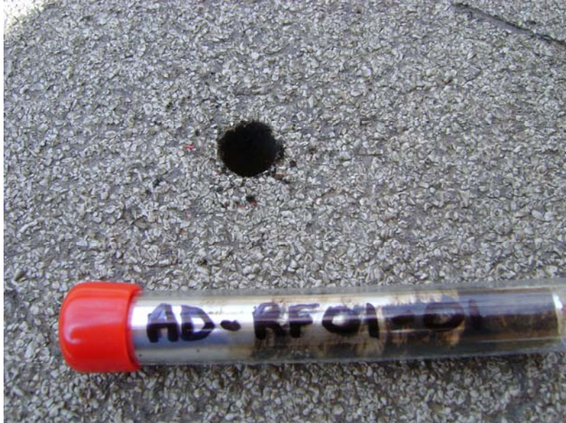
Photo 3 – View of roofing shingles containing 15% Chrysotile.
